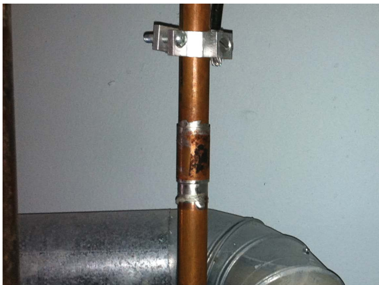
FIGURE 1-3: Copper water pipe soldering
